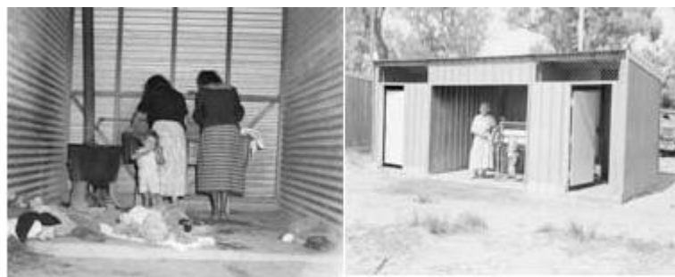
Wash room facilities at a Native Reserve in Merredin, 1960s
